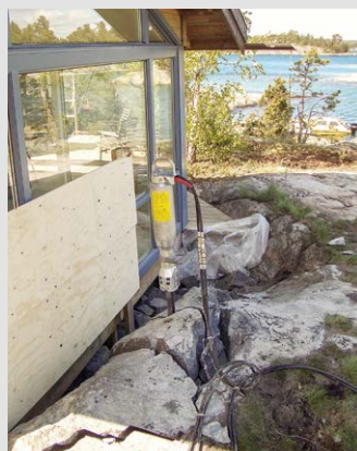
Demolition of rock and natural stone
