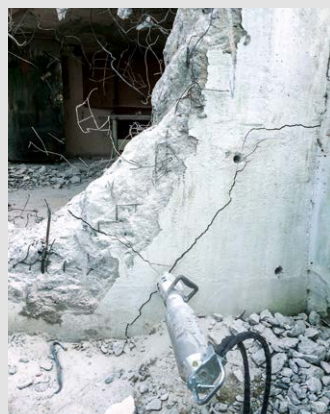
Demolition of concrete and reinforced concrete
